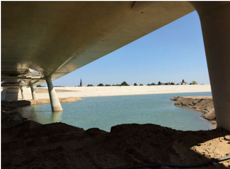
11 Room for the River project at Nijmegen under construction
