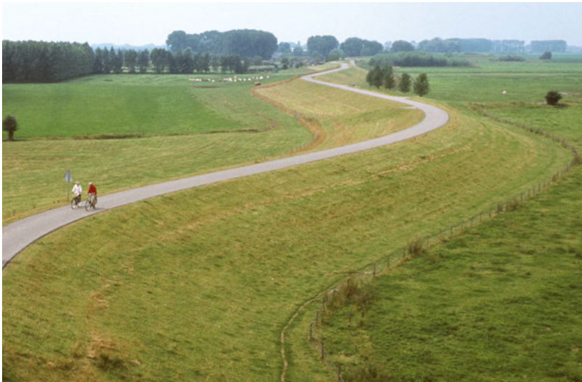
9 Dike reinforcement Afferden-Dreumel, H+N+S Landscape Architects
