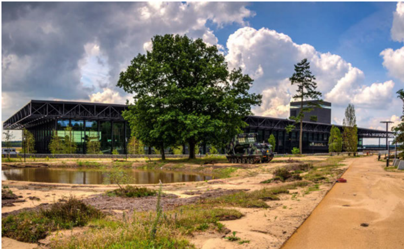
22 Recently constructed nature reserve at Soesterberg National Military Museum, heathland development and bomb crater
